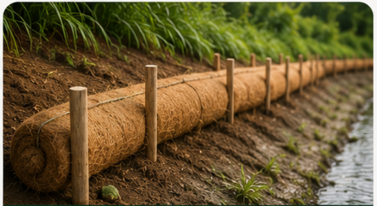
STRUCTURAL COIR LOG BARRIERS & FASCINES
